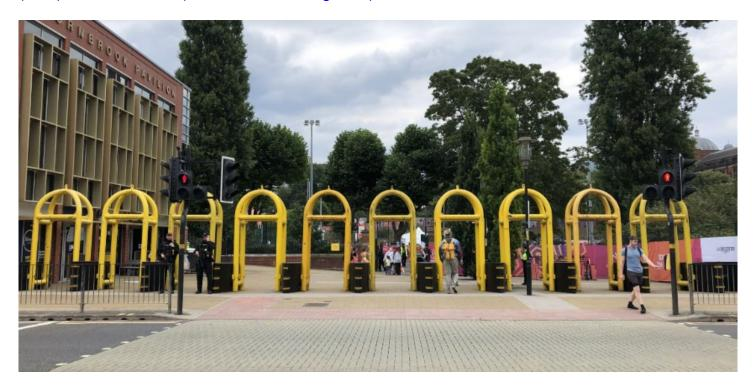
The National Barrier Asset (NBA) consists of various types of vehicle security barriers and protective security fencing to prevent/mitigate Vehicle Borne terrorist attacks (Vehicle Borne Improvised Explosive Device (VBIED) or Vehicle as Weapon (VAW)) against the public at Venues and Public Spaces.
