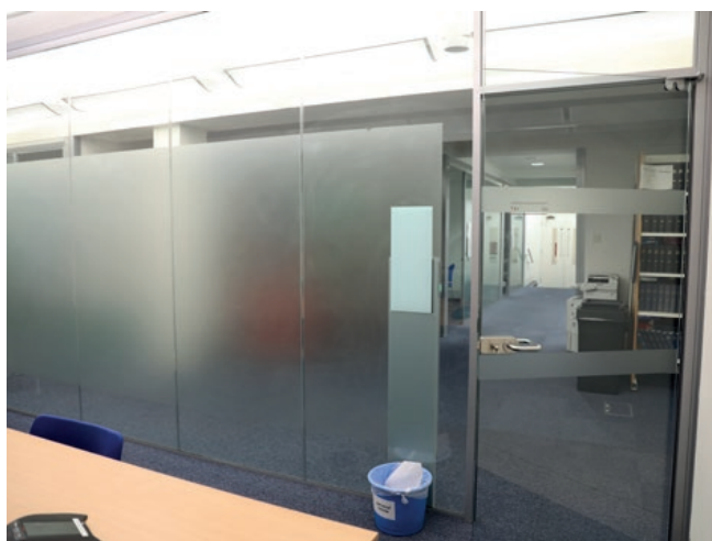
Figure 6: Frosted internal glazing
