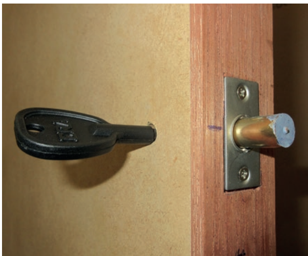
Figure 7: Low-cost key-operated door bolt retrofitted to a hardwood timber door
