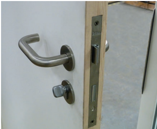
Figure 4: Bolt operated by a thumb-turn that needs little dexterity, is operated by a single, reversible action and requires no additional equipment
