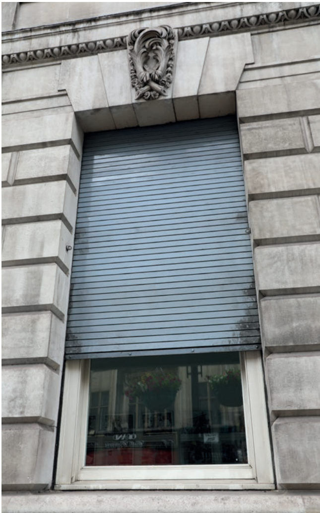
Figure 15: Roller shutter covering a window
